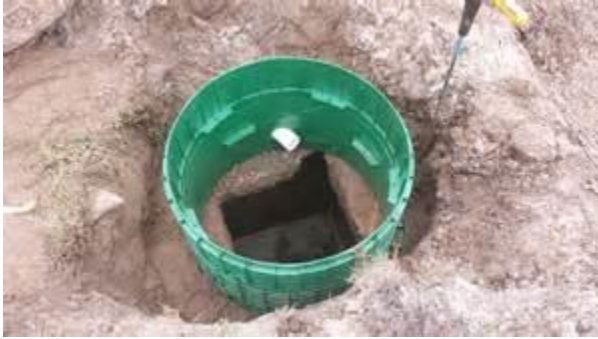
Installation of a plastic riser on an existing septic tank
