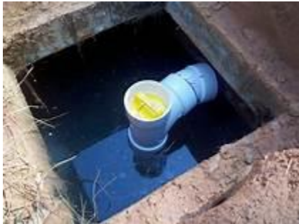
Effluent filter retrofitted to an existing concrete septic tank
