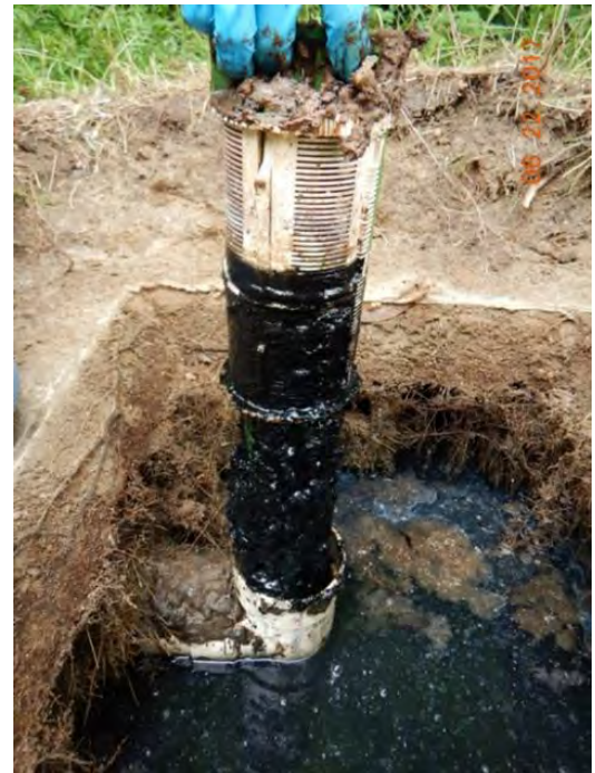
Illustration 2 – Clogged Effluent Filter
