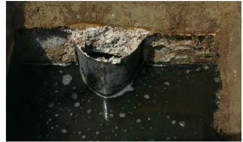
Illustration 1 - Concrete Corrosion Around Outlet Baffle
